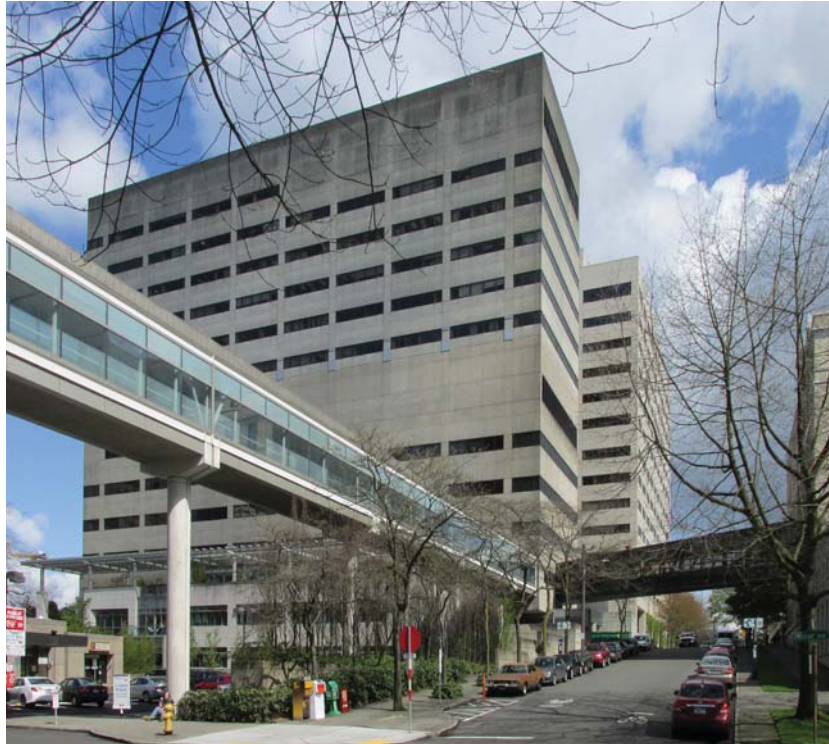
Existing Marion skybridge
